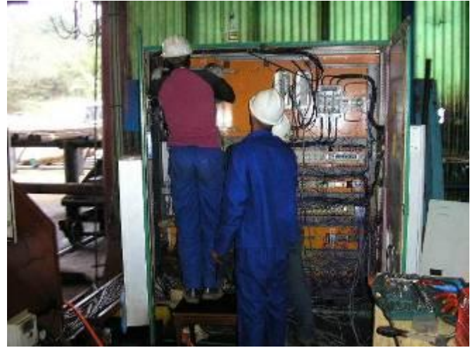
Figure 18: The maintenance people build anything, it serves as their training.
