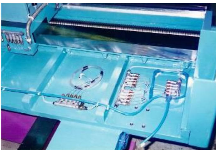
Figure 13: Dossier lubrication system with units and air withdrawal
