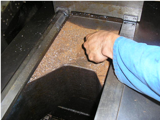
Photo: Dan, one finds the rust under all covers, almost like in Angola! So you decide to unscrew many sheets.
