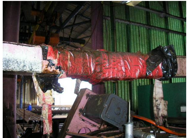
Photo 2: Here you have prevents water from running into the CNC, nevertheless was always wet. It looks like a large amount of condensation. The aircon was always running at full speed.
