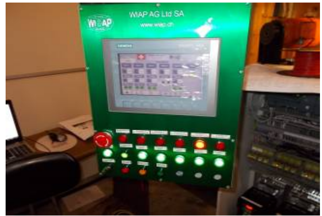
The panel in the final assembly phase. WU5130s
